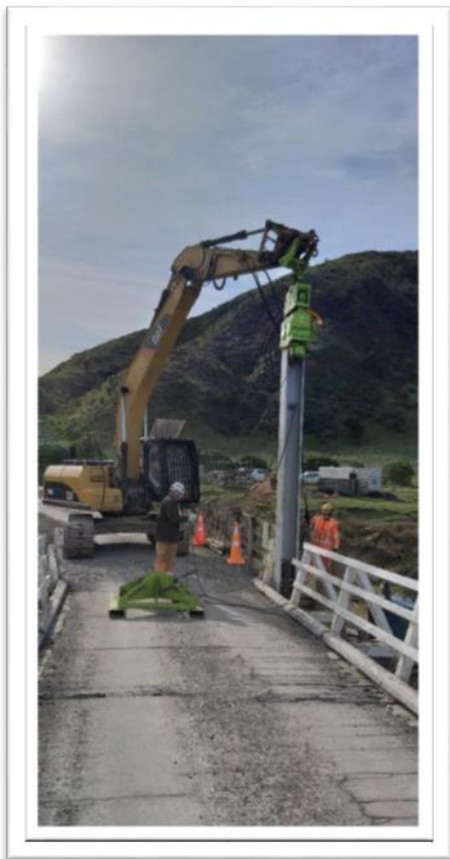
Pile driving Tora farm Settlement bridge.
